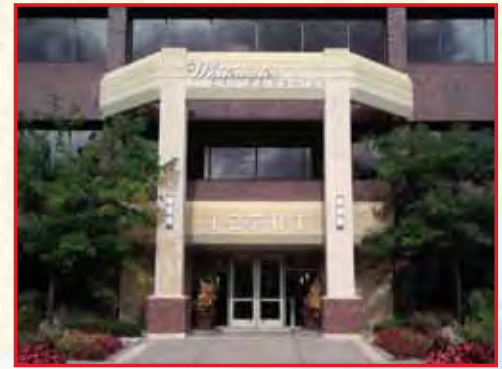
The Whitewater Office Center, the new home of FaithSearch International.
